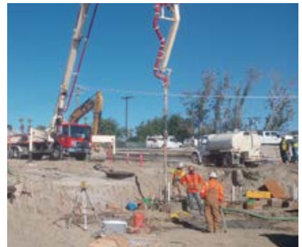
Crews placing concrete into the steel cage around the steel pile.
