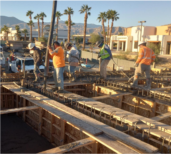
Crews placed 840 yards of concrete on the northbound/western bridge interior.
