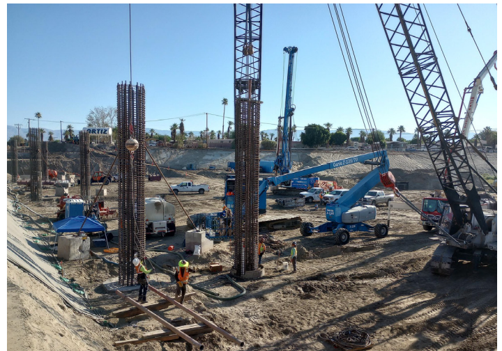
Crews performing the placement process and rebar work for the 60-inch rebar cage columns, which is part of bridge foundation work.
