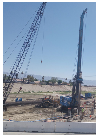
Crews receiving the next set of bridge support foundation cages. These rebar cages measure 5-feet by up to 110-feet-long and will be set into the ground near the current bypass roadway to eventually support the new northbound eastern bridge span.
